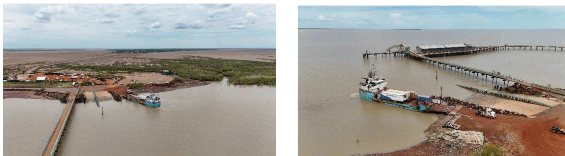
Figure 3: Images showing the BLF and commercial slipway
